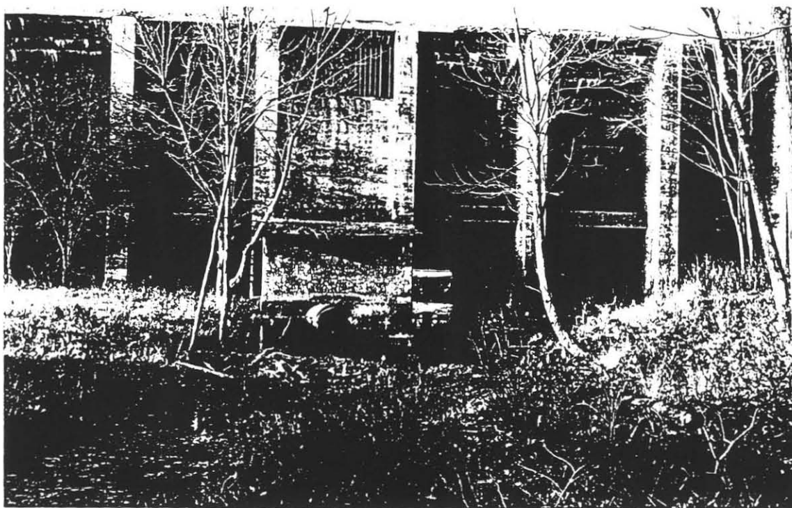
Figure 5. The Million-Dollar Dam looking northwest from the reservoir outlet.
